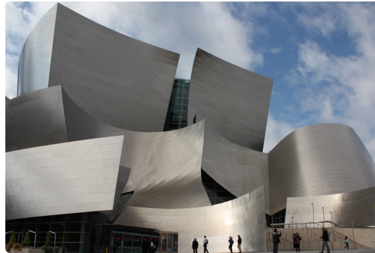
#4 | Frank Gehry | Walt Disney Concert Hall | 2003 | stainless steel exterior Los Angeles, CA
